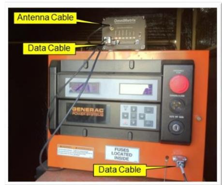
Data Cable and Antenna Cable Connections.
