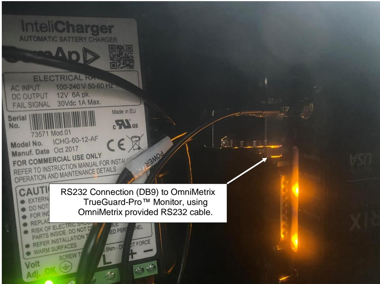
RS232 Connection (DB9) to OmniMetrix TrueGuard-Pro™ Monitor, using OmniMetrix provided RS232 cable.
